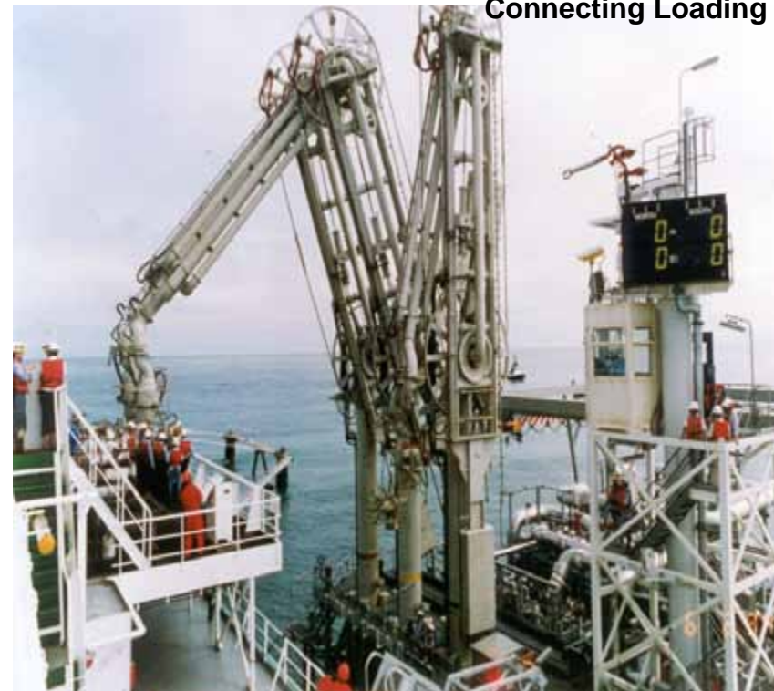
Connecting Loading Arms
